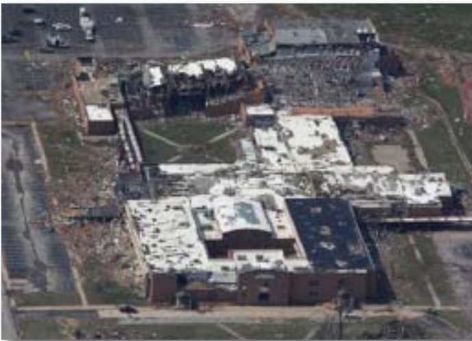
Joplin High School after the tornado.
