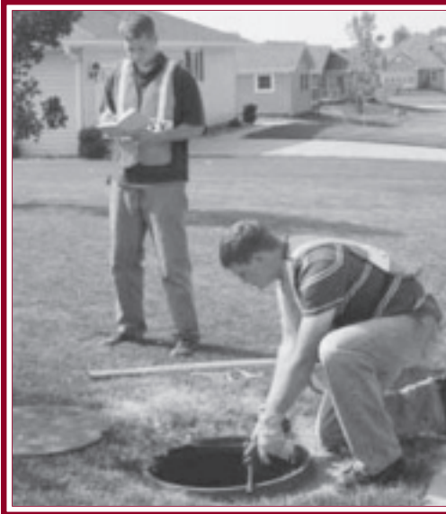
Midland GIS Solutions field technicians use V-Depth equipment to obtain accurate invert depths for a sanitary sewer project. Using this eliminates dipping each manhole with a conventional level rod.
